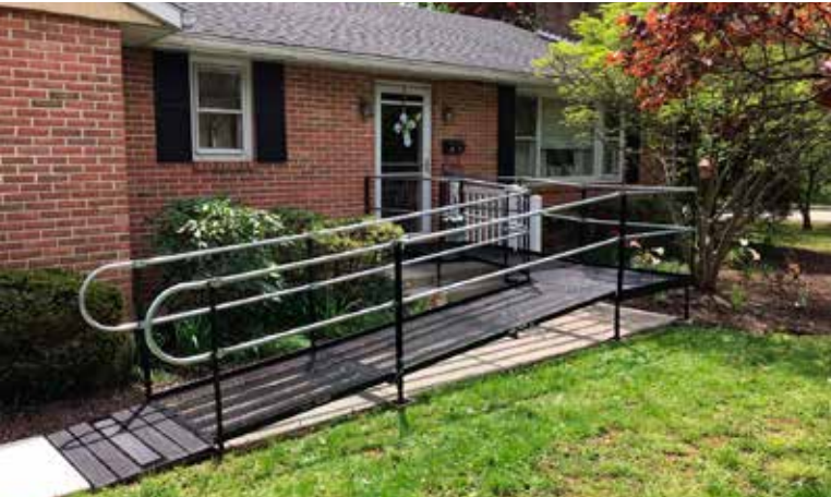
Residential Wheelchair Ramps
